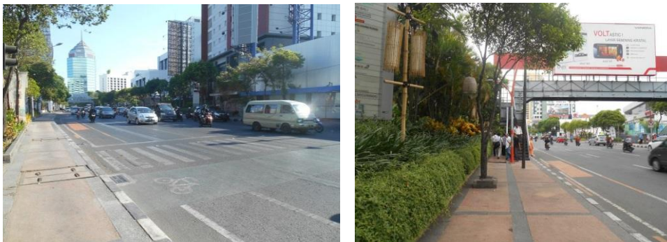
Figure 9. Condition of Crossing Facilities in Observed Pedestrian Pathways Source: Primary Survey, 2014
