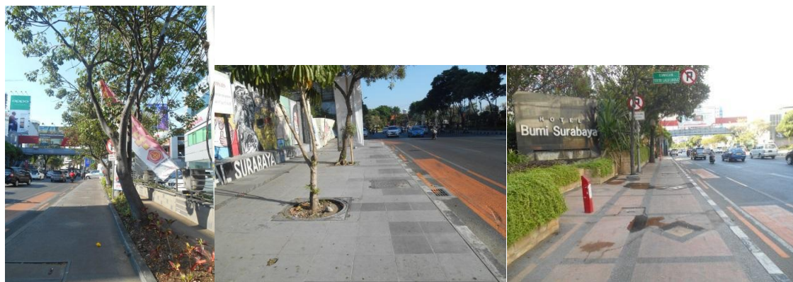
Figure 3. Sidewalk on the East and West Sides of the Road (Source: Primary Survey, 2014)
