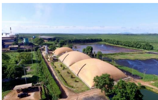
Gambar 2. Instalasi methane capture pada kolam limbah cair pabrik kelapa sawit ( https://anj-group.com/en/renewable-energy )
