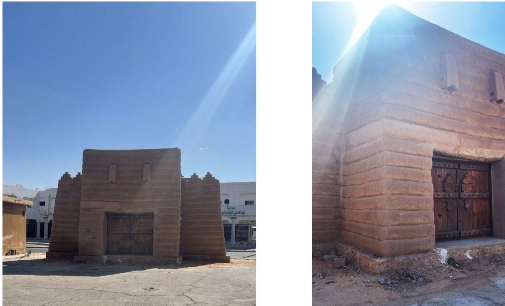
Fig. 3. West Gate, Buraydah, Al Qassim
