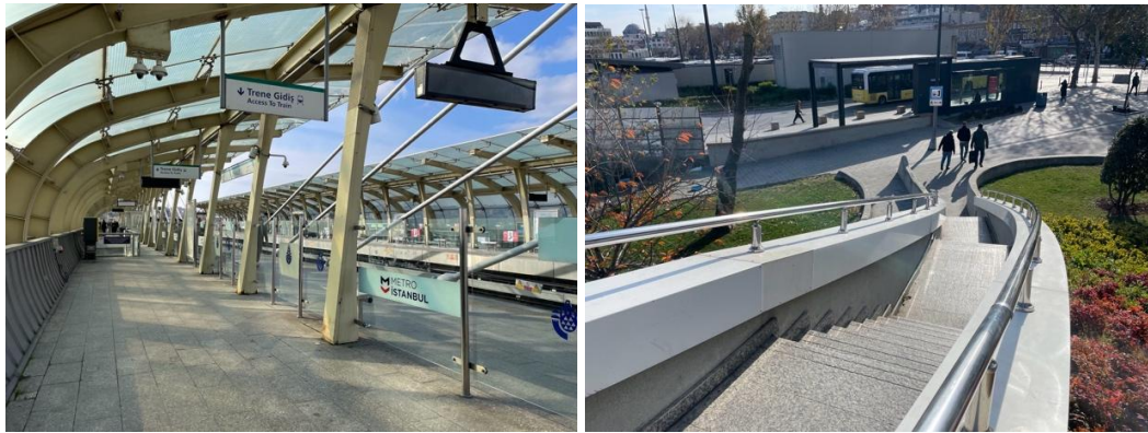
Fig. 3. Pedestrian Access and Underutilized Public Spaces on Haliç Metro Köprüsü
