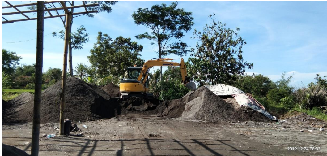
Figure 1. One of the sand depots in Keningar Village (Author Documentation, 2019)
