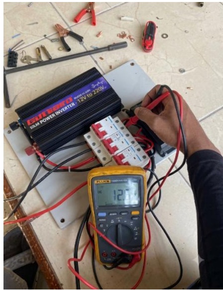
Fig. 6. installation and assembly of materials
