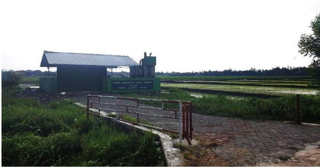
Figure 1. Waste Treatment Facility (TPS) of Desa Paulan
