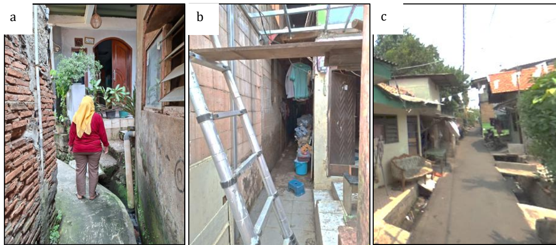
Fig. 2 (a) Narrow access roads within the residential area; (b) Narrow alleyway adjacent to the residence of a participant with an intellectual disability; (c) Wide open drainage channel near the residence of a participant with visual impairment.
